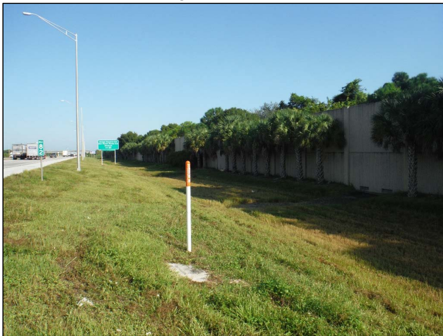
Figure 7 – Berm, Ditch, Buried Utilities, and Sound Wall Illustrated along Northbound SR 9/I-95 South of Hood Road, Facing North-Northwest
